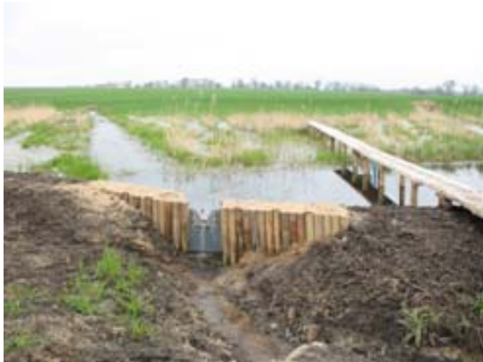
Pond outlet and gauging weir
