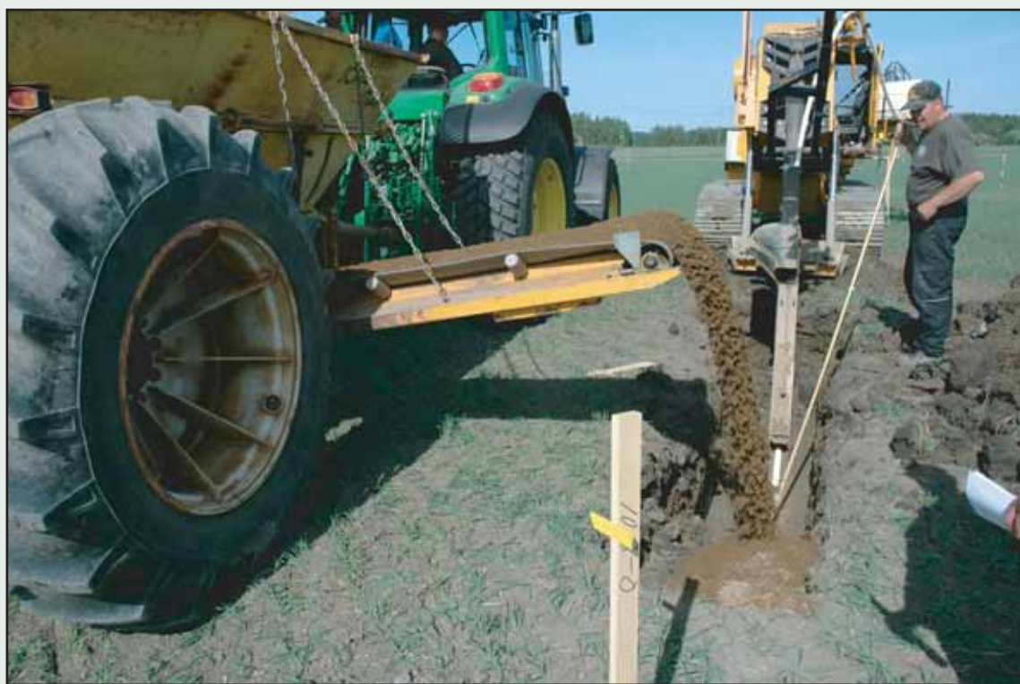
In method I the additional drainage was done with a drainage trencher, plastic pipe and gravel was used as envelope material.
