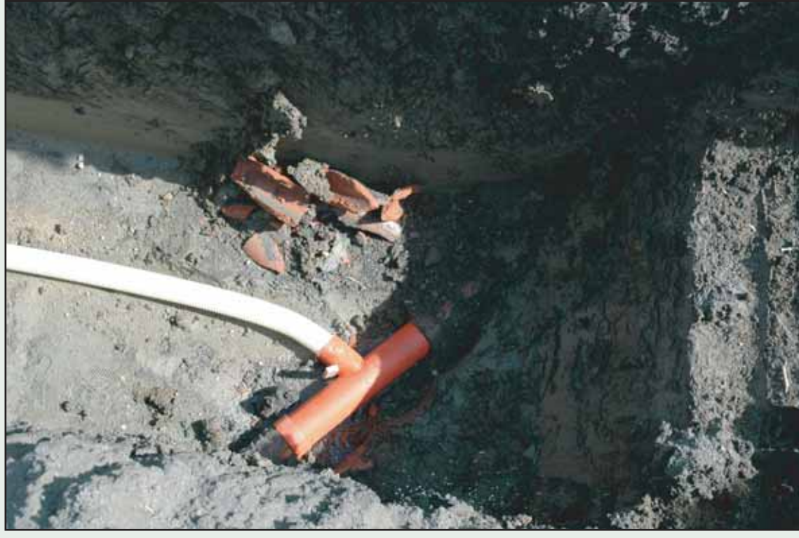
The new pipes were laid between the old ones and connected to the existing collector.
