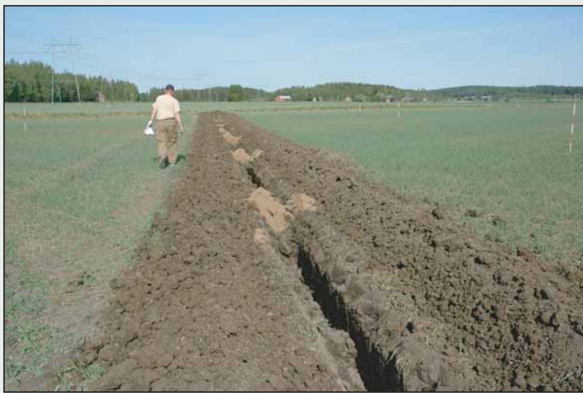
Gravel was filled to the top (blind inlet) every 8 meters. The trenched soil was left to dry for a week after which it was used to fill up the trench.
